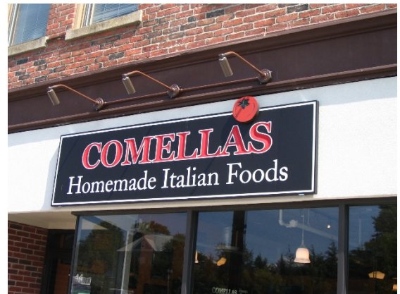
A good example of exterior lighting of façade signs using gooseneck lights.
